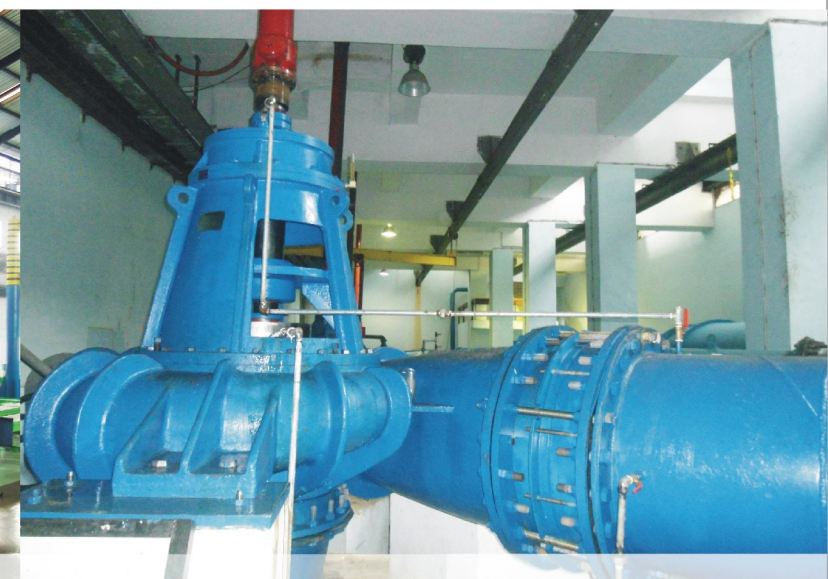
TG CFV Pump Installation
