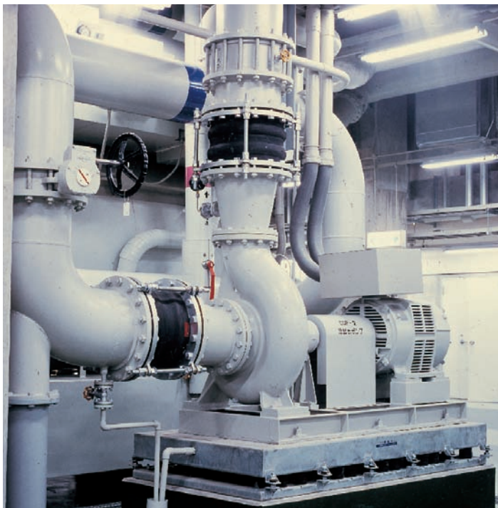
Cooling Water Pump / District Heating and Cooling Plant
