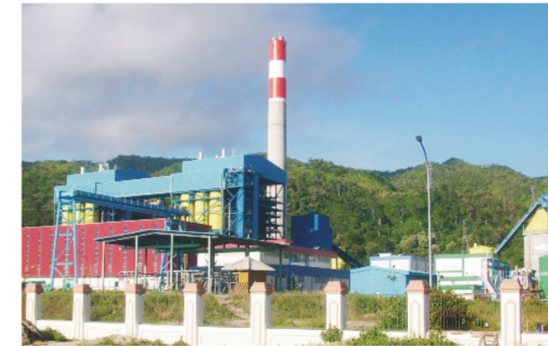
Tarahan Steam Power Generation, Indonesia
