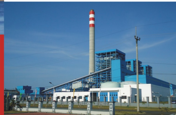
Muara Karang Combined Cycle Power Plant, Indonesia
