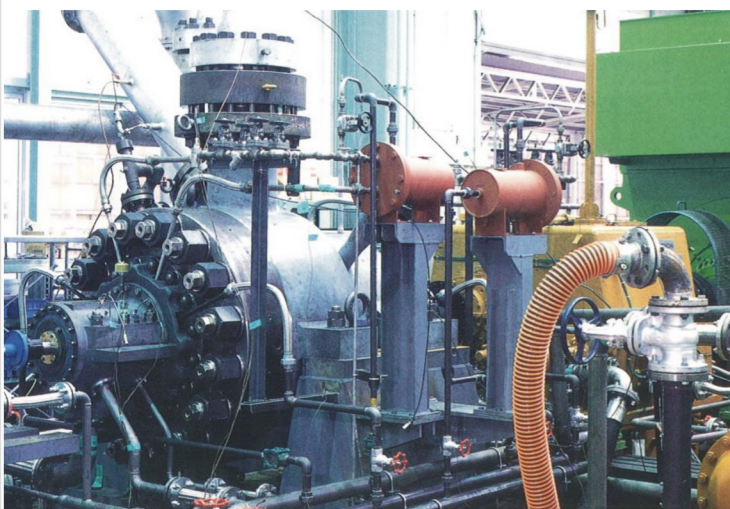
MHB Barrel type Boiler Feed Pump , Having 100 % load capacity (for Elbistan - B P/S. 360 MW) Turkey.
